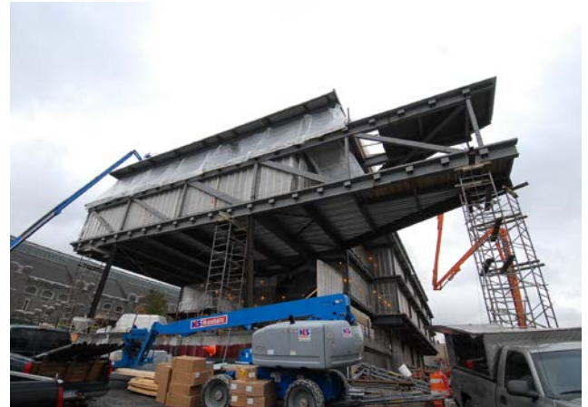
CIS Building Site – southwest facade
