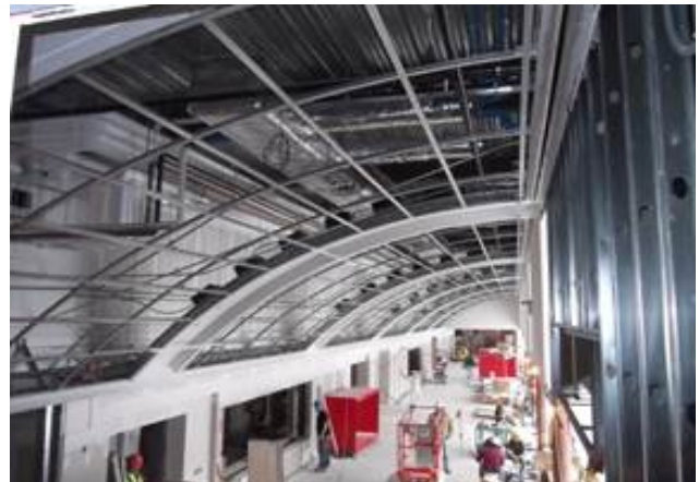
12/28/12 – Stocking Hall-Gallery - looking west from the stair landing
