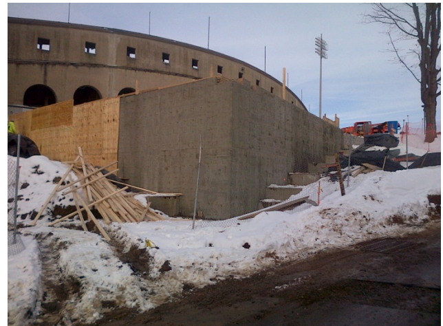
1/8/13 – Concrete foundation walls
