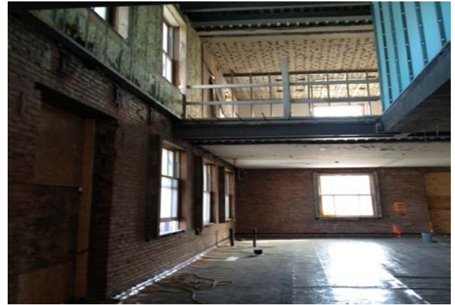
Fernow Hall Basement – view into future Stair B.
