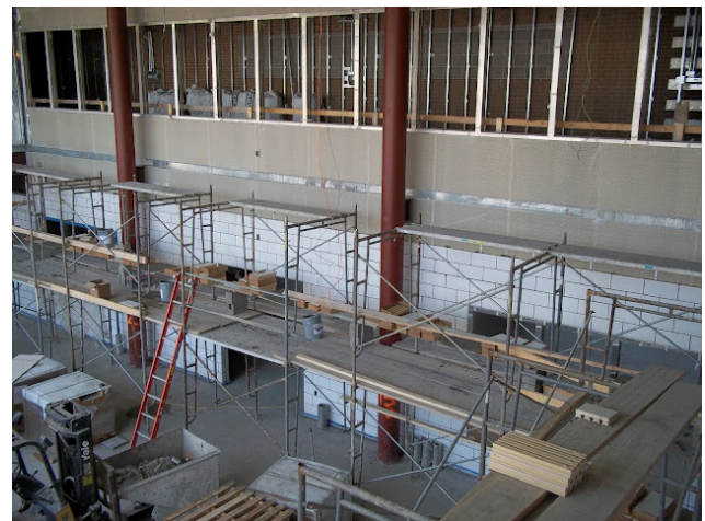
3/20/12 – View of Cornell Dairy Plant looking South.
